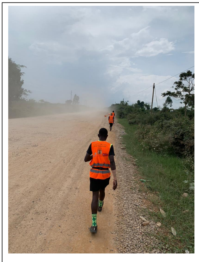
The team walking through the dusty and stoney road under construction in Mityana.
